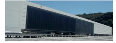
Solar cell system integrated into the building envelope
