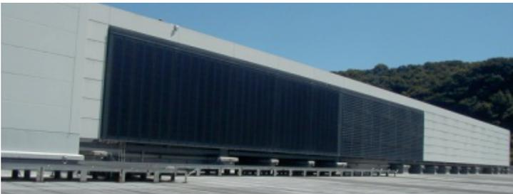
Solar cell system integrated into the building envelope
