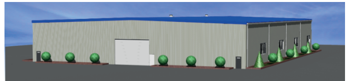
Image of Pretreatment facility
