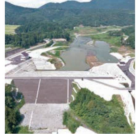
Ichinoshinden Dam [Niigata, 2019]
