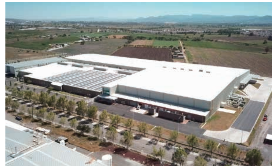
Mitsubishi Electric Querétaro Factory [Mexico, 2020]
