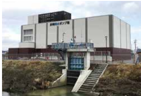
Harisaki rain water pumping station [Aichi, 2014]
