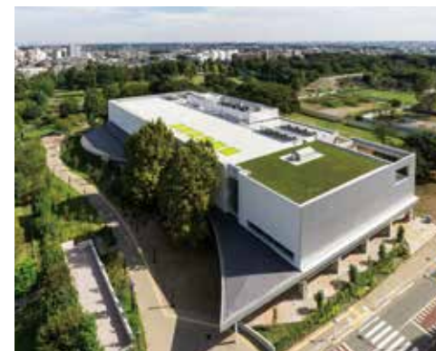
Tokyo Metropolitan Tama Library [Tokyo, 2016]
