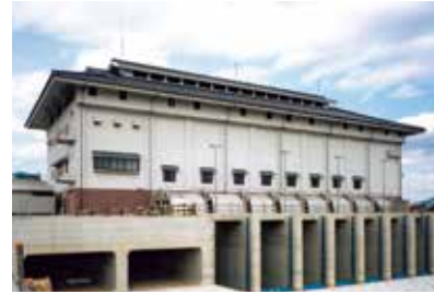
Oguraike Drainage Station / Sluiceway [Kyoto, 2004]
