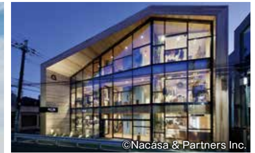
G Building Jiyugaoka 01 B-Bld. [Tokyo, 2016]
