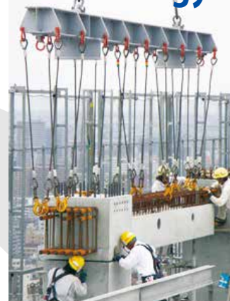
Construction using the precast concrete method (an example of the FHRC construction method)
