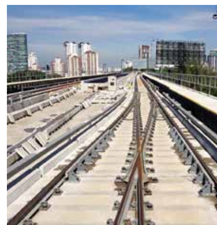
KVMRT Project [Malaysia, 2016]
