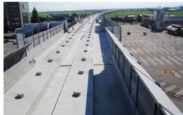
Imizu Ima Kaihotsu Viaduct, Hokuriku Shinkansen [Toyama, 2012]
