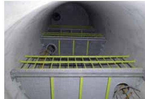
Zasshonokuma Dai 6 rain water main line [Fukuoka, 2015]
