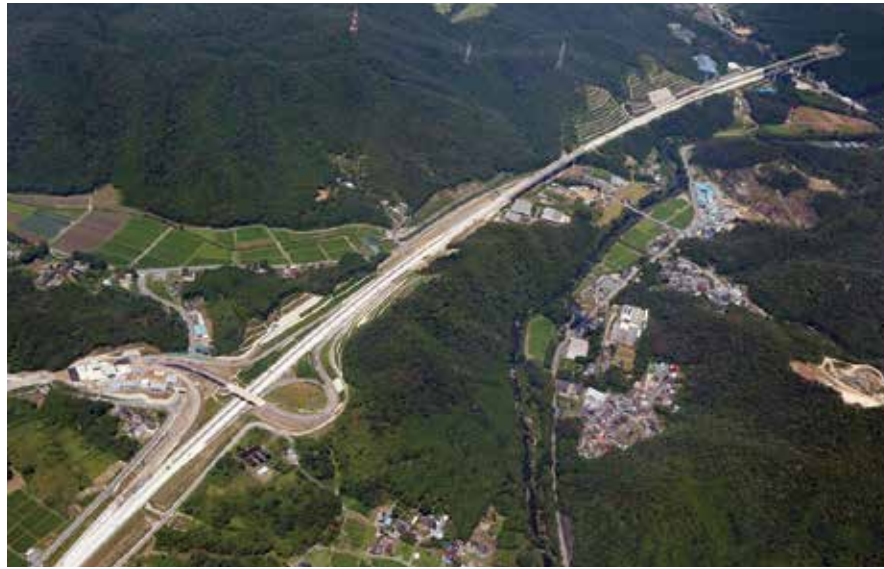
Nukata IC, Dai 2 Tomei (Tokyo-Nagoya) Expressway [Aichi, 2015]
