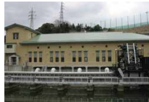
Ryoso water Dai 1 irrigation pumping station [Chiba, 2005]
