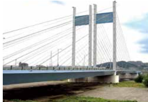
Koremasa Bridge [Tokyo, 2017]
