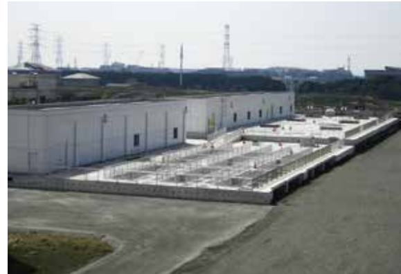
Kimitsu Futtsu Sewage treatment plant [Chiba, 2014]
