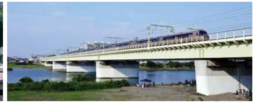
Tamagawa Bridge [Tokyo, 2008]
