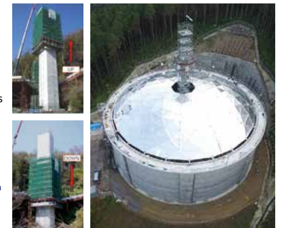
Aluminum dome roof installation example
