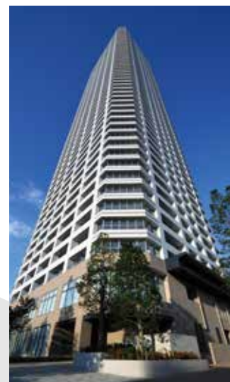
Construction example using reinforced concrete high-rise technology
