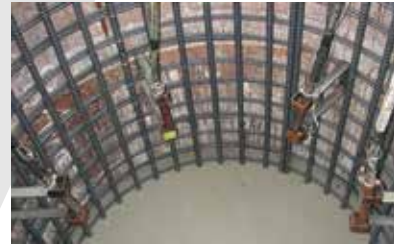
Pile head vibrator installation
