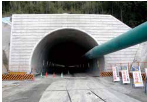
Kasamori Tunnel, Ken-O Expressway [Chiba, 2010]
