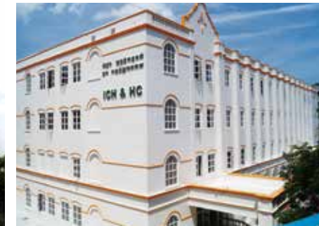
Chennai Children's Hospital [India, 2016]
