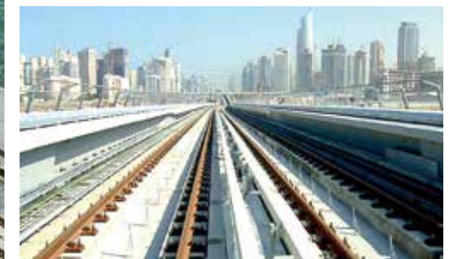
Dubai Metro (Red Line) [United Arab Emirates, 2009]
