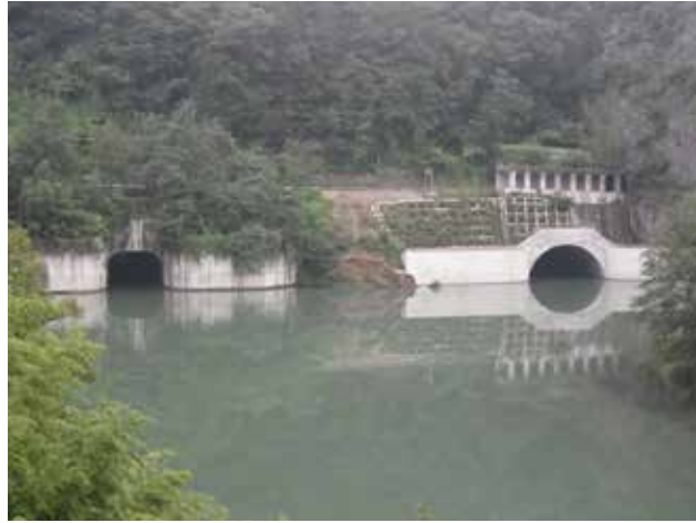
Saigawa River Tunnel [Nagano, 2014]
