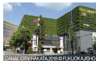
Left: Co-Op Kyosai Plaza (Tokyo) Received the Ministerial Prize for Green Walls at the 15th Rooftop and Wall Special Green Technology Competition in 2016. Above: Canal City Hakata, East Bld. (Fukuoka) Received the above award in 2013.
