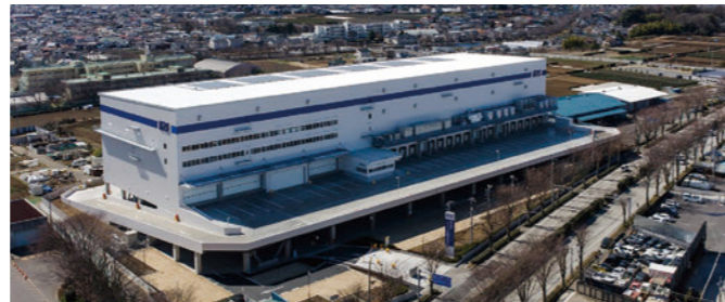
Kyuso Distribution System Tokorozawa Distribution Center [Saitama, 2014]
