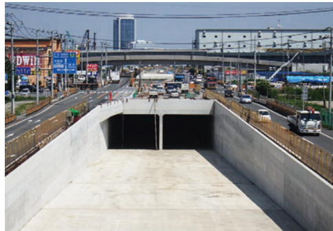
Toda Crossing Underpass [Kanagawa, 2016]
