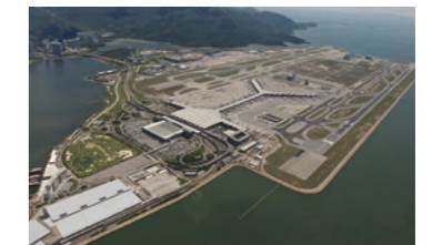
Hong Kong International Airport
