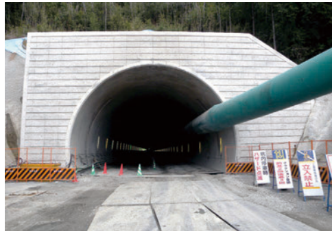
Kasamori Tunnel, Ken-O Expressway [Chiba, 2010]
