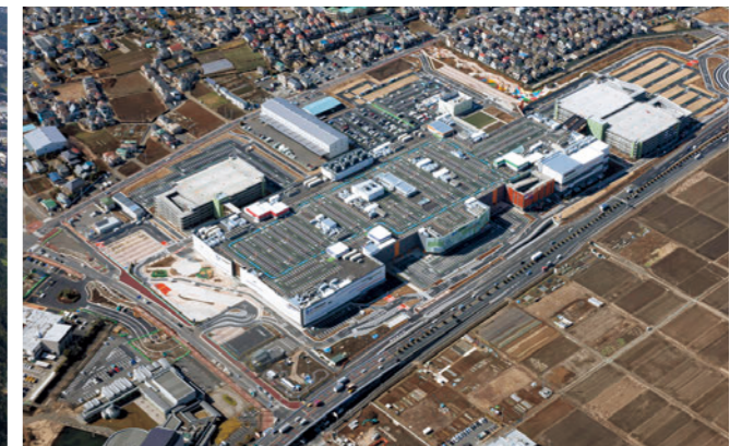
Development of infrastructure, Mitsui Shopping Park LaLaport Fujimi [Saitama, 2015]
