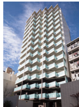
The Parkhouse Yanaka Dokanyama Residence [Tokyo, 2017]
