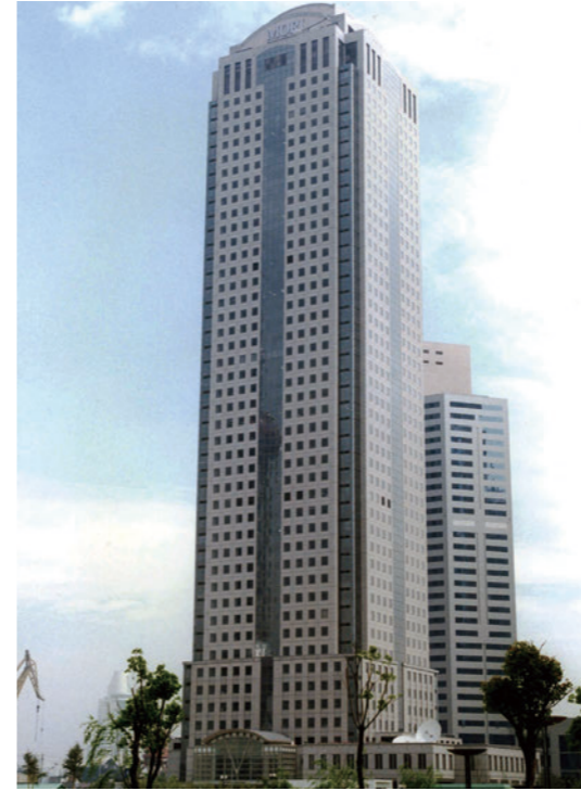
Hang Seng Tower [China, 1998]
