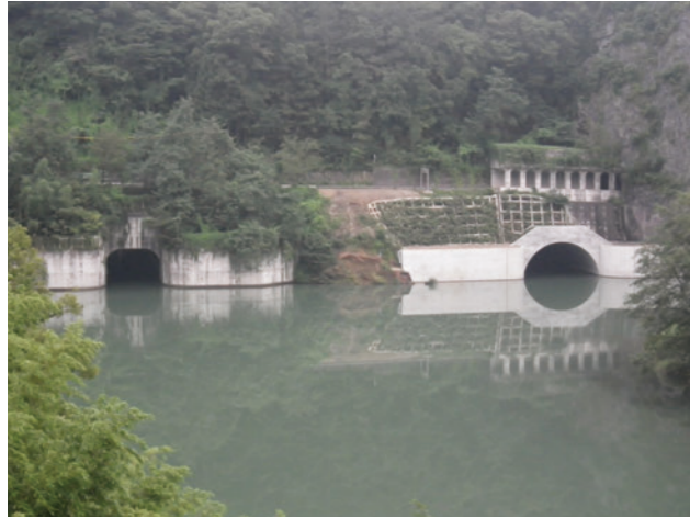
Saigawa River Tunnel [Nagano, 2014]
