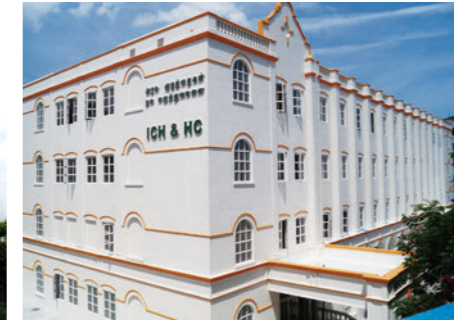
Chennai Children's Hospital [India, 2016]
