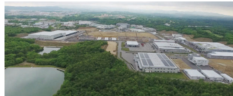
Hokusetsu Sanda Dai 2 Techno 2nd period construction [Hyogo, 2016]
