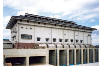
Oguraike Drainage Station / Sluiceway [Kyoto, 2004]
