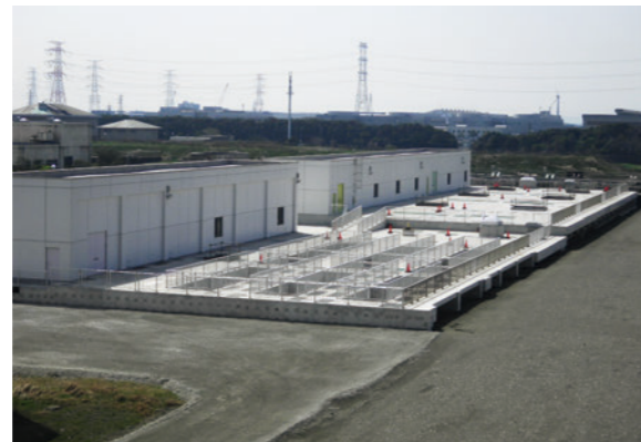
Kimitsu Futtsu Sewage treatment plant [Chiba, 2014]
