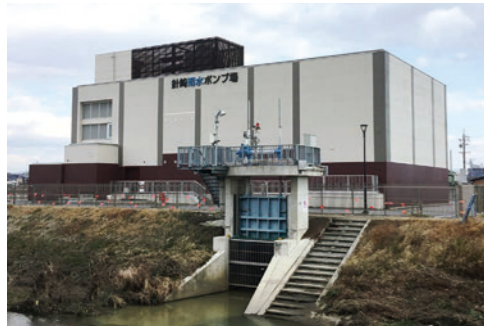
Harisaki rain water pumping station [Aichi, 2014]
