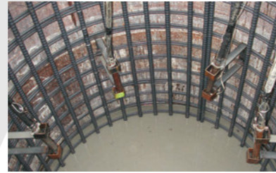
Pile head vibrator installation
