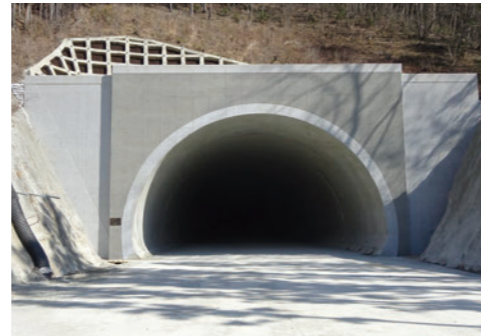
Enbuchi Tunnel, National Route 115 [Fukushima, 2017]
