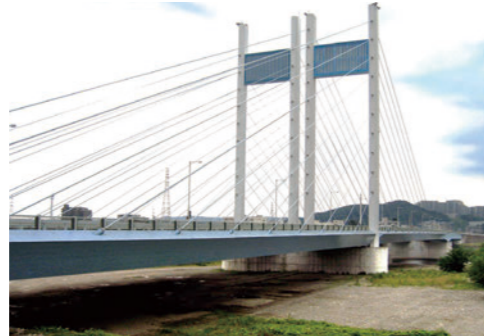
Koremasa Bridge [Tokyo, 2017]
