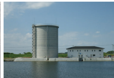
Inba-numa 2nd period agricultural water conservatory project Sougokita pumping station [Chiba, 2016]
