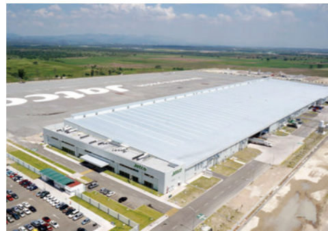
The new 2nd Plant, JATCO Mexico, S.A. de C.V. [Mexico, 2014]
