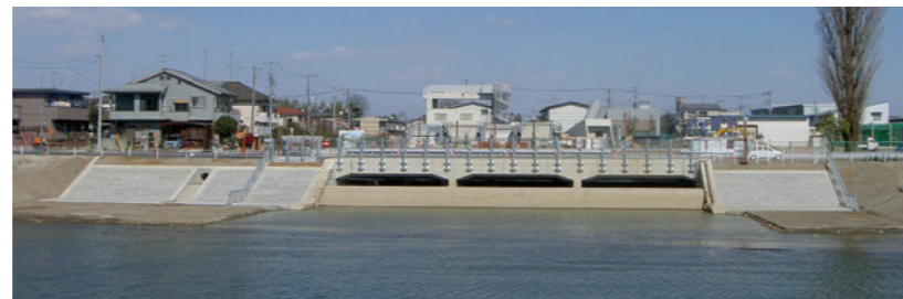
No.5 Vertical shaft inflow facility, Outer Underground Discharge Channel [Saitama, 2007]
