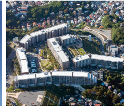
The Parkhouse Oppama [Kanagawa, 2015]
