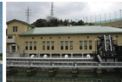
Ryoso water Dai 1 irrigation pumping station [Chiba, 2005]
