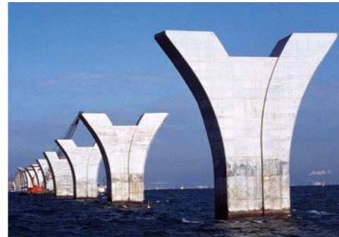
Bridge pier part, Tokyo Wan Aqua-Line Expressway [Chiba, 1994]
