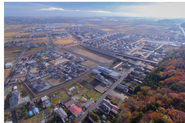
FY 2013 Act to Assume Debts No. 1, Urban area around Shin Yamashita Station outside of maintenance construction [Miyagi, 2016]
