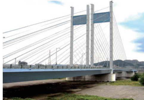
Koremasa Bridge [Tokyo, 2017]
