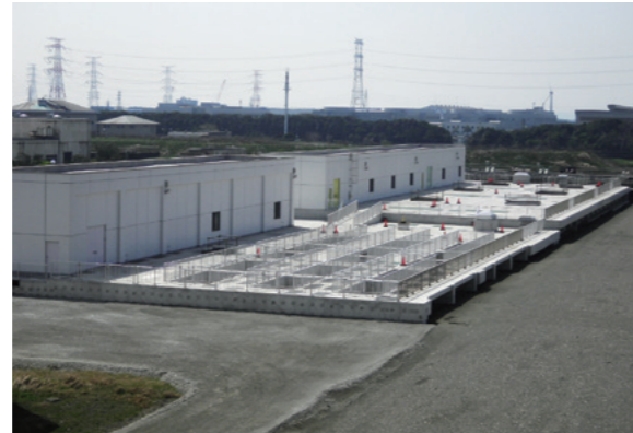
Kimitsu Futtsu Sewage treatment plant [Chiba, 2014]
