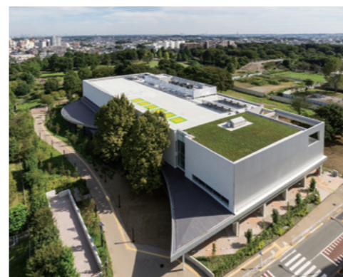
Tokyo Metropolitan Tama Library [Tokyo, 2016]
