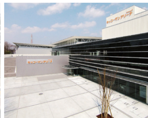
Kikkoman Arena (Nagareyama Municipal Gymnasium) [Chiba, 2015]
