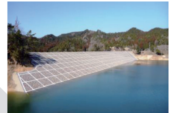
Example of fill dam embankment repair using the stabilized muddy soil embankment method
