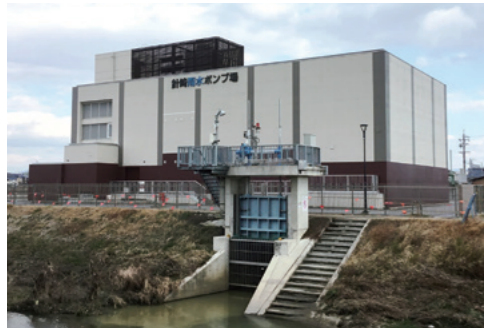
Harisaki rain water pumping station [Aichi, 2014]
