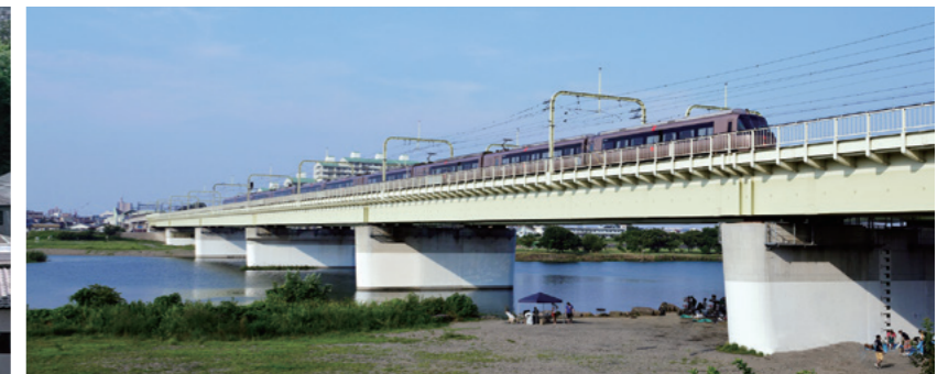
Tamagawa Bridge [Tokyo, 2008]
