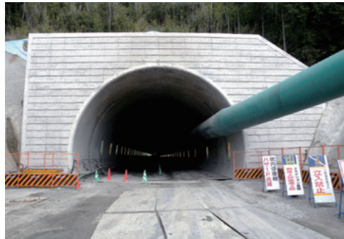
Kasamori Tunnel, Ken-O Expressway [Chiba, 2010]
