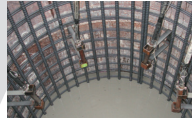
Pile head vibrator installation
