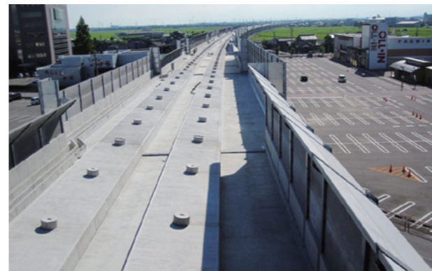
Imizu Ima Kaihotsu Viaduct, Hokuriku Shinkansen [Toyama, 2012]
