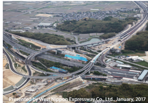
Presented by West Nippon Expressway Co., Ltd., January, 2017 Yawata Junction, Shin-Meishin Expressway [Kyoto, 2017]
