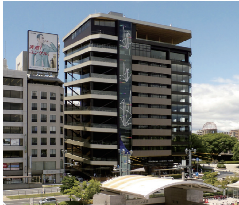
Orizuru Tower [Hiroshima, 2016]
