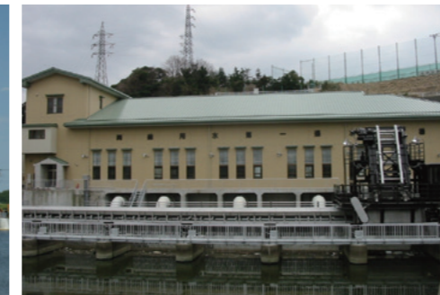
Ryoso water Dai 1 irrigation pumping station [Chiba, 2005]
