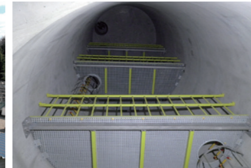
Zasshonokuma Dai 6 rain water main line [Fukuoka, 2015]
