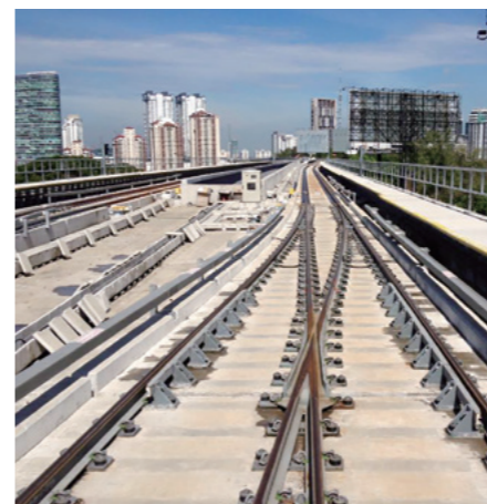
KVMRT Project [Malaysia, 2016]
