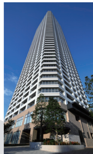
Construction example using reinforced concrete high-rise technology
