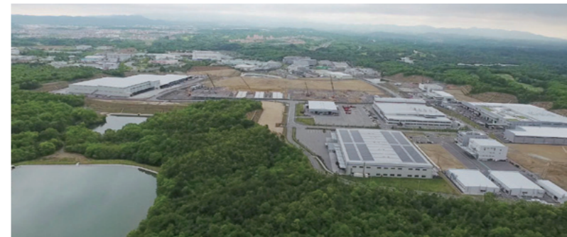
Hokusetsu Sanda Dai 2 Techno 2nd period construction [Hyogo, 2016]
