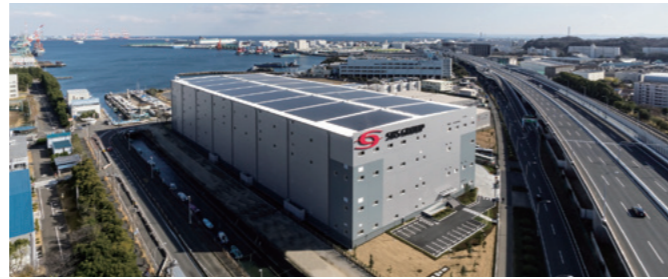
SBS Logicom Shin Sugita Logistics Center Branch [Kanagawa, 2016]
