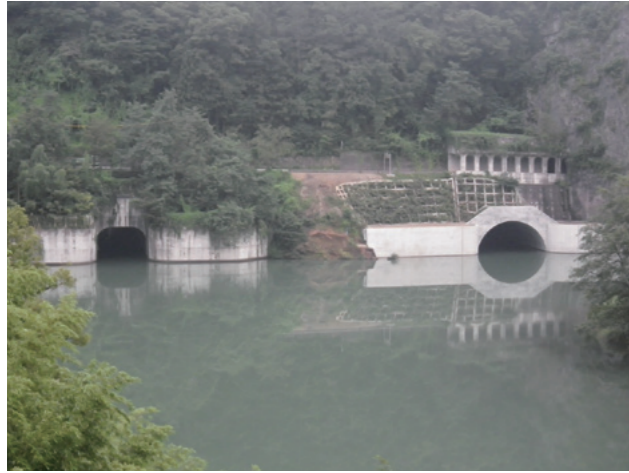
Saigawa River Tunnel [Nagano, 2014]
