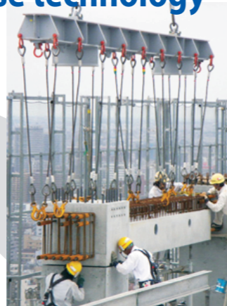
Construction using the precast concrete method (an example of the FHRC construction method)
