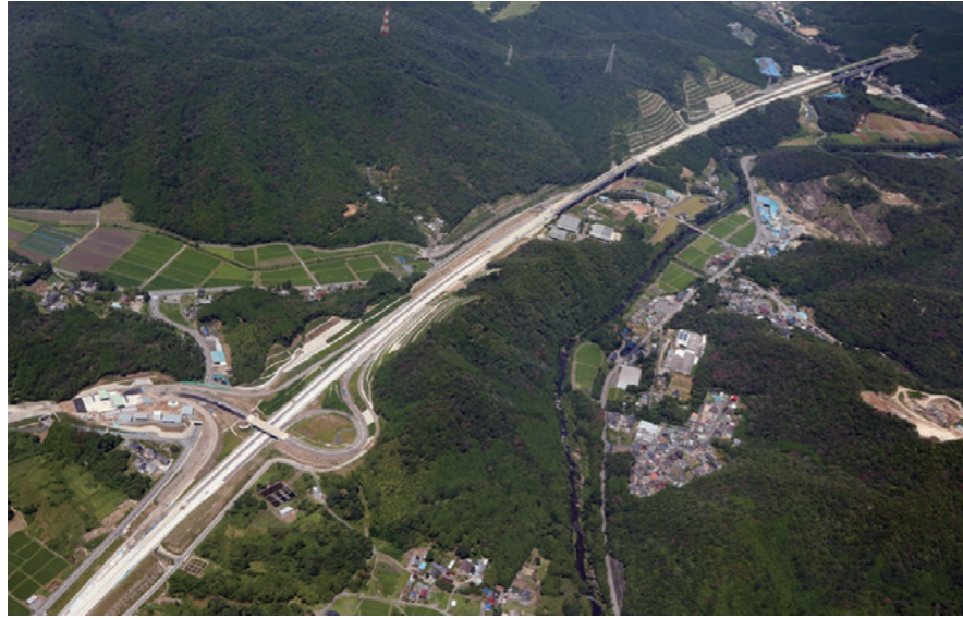
Nukata IC, Dai 2 Tomei (Tokyo-Nagoya) Expressway [Aichi, 2015]
