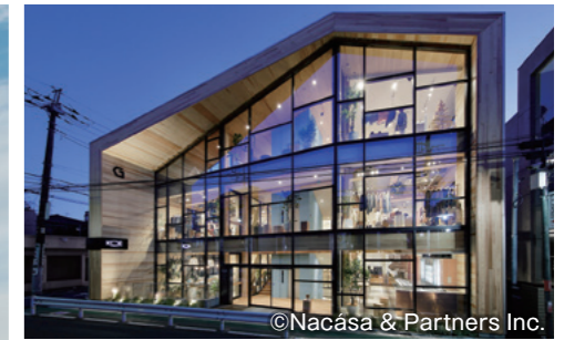
G Building Jiyugaoka 01 B-Bld. [Tokyo, 2016]
