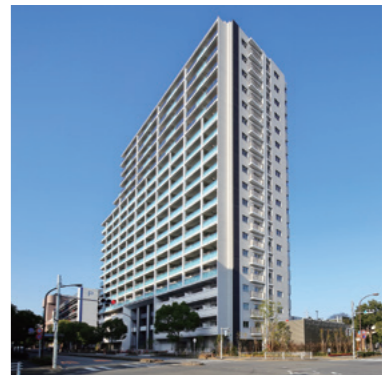
The Parkhouse Tama Center [Tokyo, 2016]
