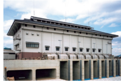
Oguraike Drainage Station / Sluiceway [Kyoto, 2004]
