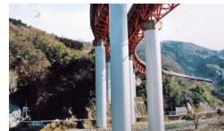
Reinforcement of Sakawa River bridge, Tomei Expressway
