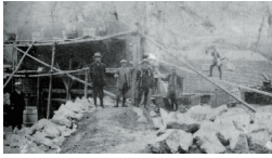
Railway laying project for Seiso Electric Railway
